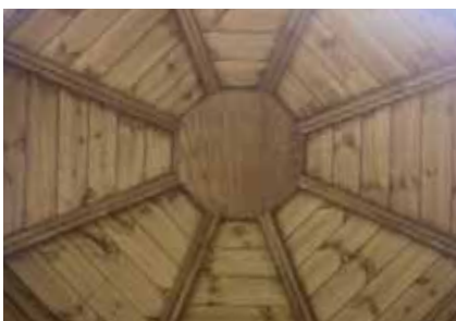
Internal roof structure
