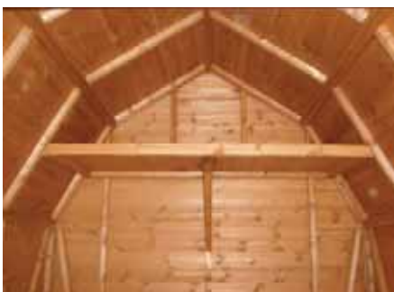
Internal roof and shelf
